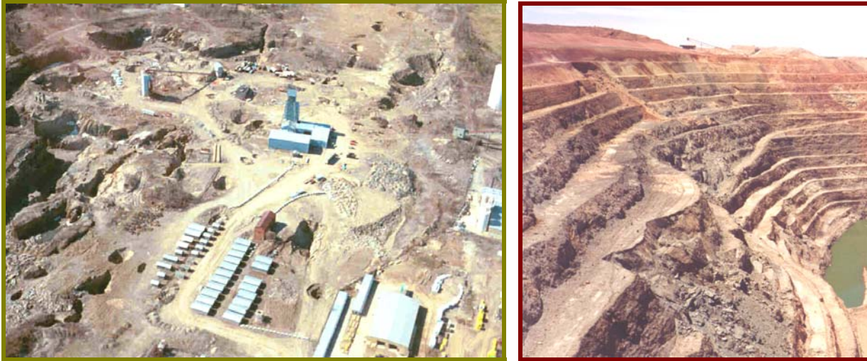
Figure 1: Ground movement associated with: 1) mine subsidence, and 2) mine pit wall instability.
